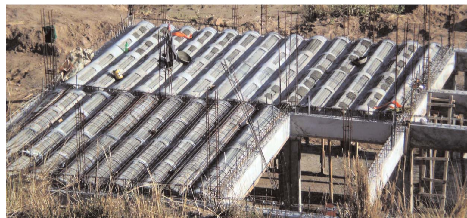
MASS Technology Roof Slab on the project near Islamabad
